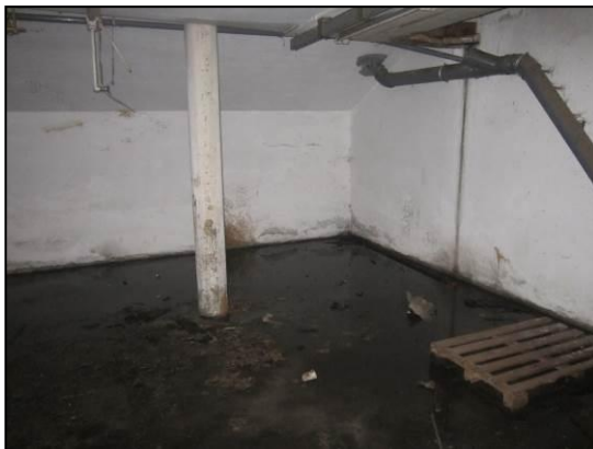
Vochtige ruimte in loods.
